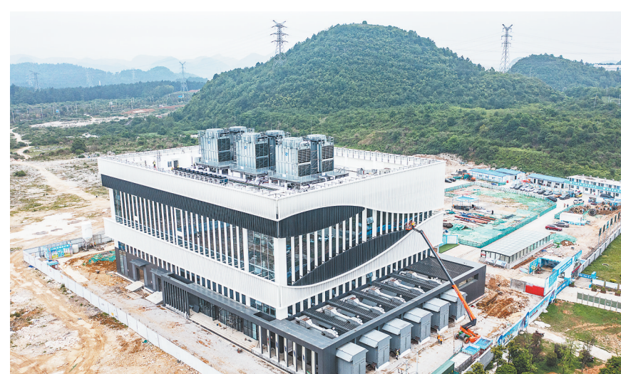
A data center under construction in Guizhou province. (PHOTO: XINHUA)
