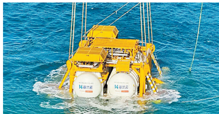
A set of data pods are lowered into the sea in Hainan. (COURTESY PHOTO)
